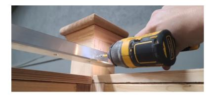
2. Place a level on the aluminum angle. Making sure the piece is leveled, screw the other end into the opposite post using the supplied 2 1/2" screws. Repeat for the second aluminum angle on the posts opposite the first.
