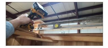
3. Screw in the first 2x2 Slat 2 1/4" from the end of the aluminum angle using the 1 5/8" screws on both ends.
