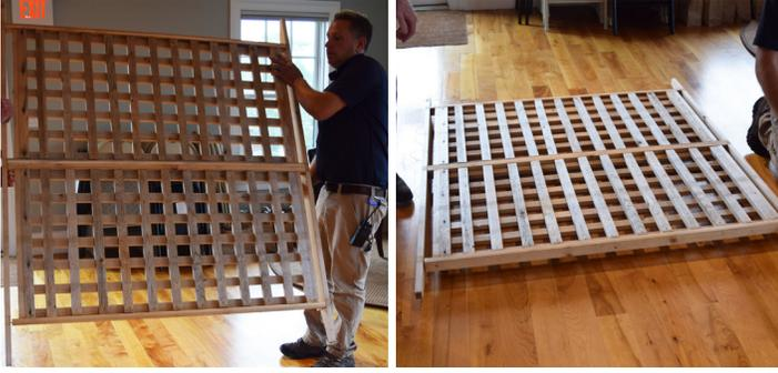
Flip the assembly over to install the 2x2 vanes.
