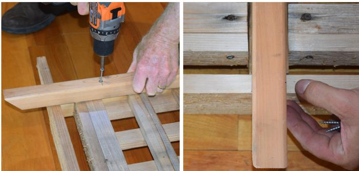
The vanes should be installed with the bevel cut facing down, one each to the right and left outside edge, one centered on the joint and the last 2 centered on the panels themselves.
