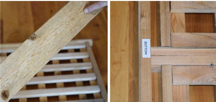
Attach the front and rear fascia boards to the ends of the roof panels. Be sure the rough side of the fascia is facing out and the "BOTTOM" sticker is facing you.
