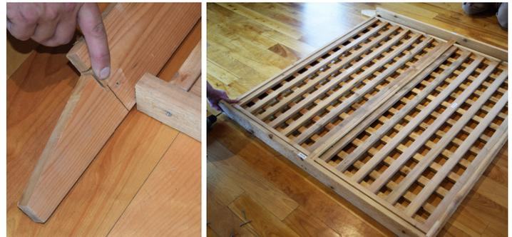
Install the fascia using 4 screws in the pre-drilled locations on both ends of your pergola top. Be sure to align the set marks on the fascia with the outer edges of the pergola top.
