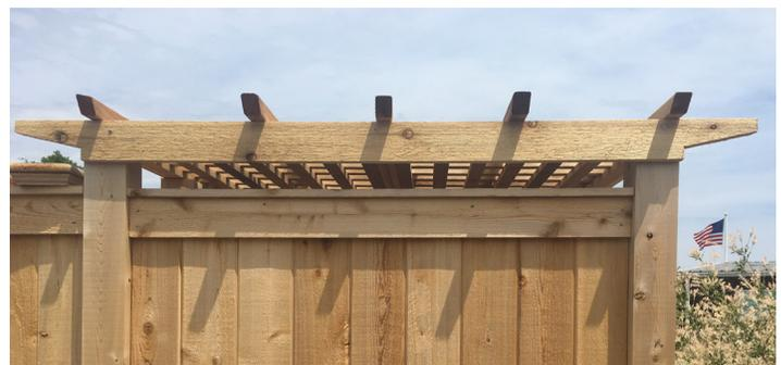
No hardware is required to attach the top. NOTE: The post caps do not get reinstalled.
