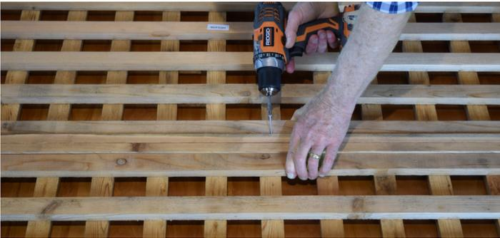
Using 3 screws from the hardware packet, attach the 2 roof panels together. You will see pre-drilled holes in the panels.
