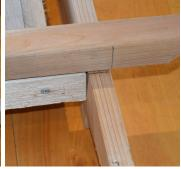
Be sure to use the predrilled holes and make sure the "UP" stickers are facing you. The vanes are marked with reference lines to allow the correct amount of overhang on each end.
