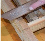
The vanes should be installed with the bevel cut facing down, one each to the right and left outside edge, one centered on the joint and the last 2 centered on the panels themselves.
