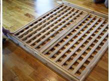
Install the fascia using 4 screws in the pre-drilled locations on both ends of your pergola top. Be sure to align the set marks on the fascia with the outer edges of the pergola top.
