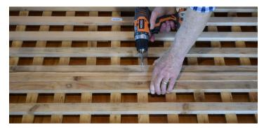
Using 3 screws from the hardware packet, attach the 2 roof panels together. You will see pre-drilled holes in the panels.
