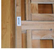
Attach the front and rear fascia boards to the ends of the roof panels. Be sure the rough side of the fascia is facing out and the "BOTTOM" sticker is facing you.
