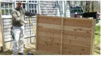
Using Timberloks<sup>™</sup> in Hardware Pack, attach a cedar post to large wall. Make sure the rainguard is on top (wider board).
