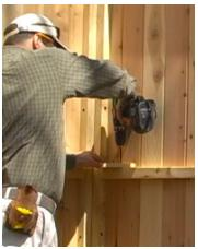
Take the small wall and attach a cedar post to it - again making sure the height from the ground matches the other 2 walls. Add the small wall.
