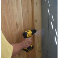
Drill with screws at an angle into the house. You can use Timberlok screws and go about 45 degrees.
