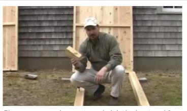
Choose your cedar posts and pick the best end for the top. Use a block or item to be reference for height for all posts. For Above Ground: Important tip the wider boards of the to remember is to decide how high off the ground you want the kit positioned. Kits are Pre-Drilled.
