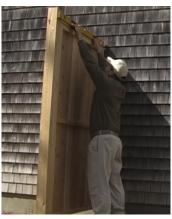
Next, attach one wall to the house. Always making sure the wall is level. Then, measure one of the walls as reference to use for the space along the back side of the house for house mounting.
