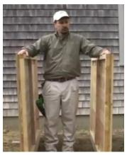
With the Pre-Drilled holes as reference use the Timberlocks<sup>™</sup> in your Hardware Pack and connect a large wall to a cedar post. Make sure the inside of the wall is flush to the cedar post. Repeat for the second large wall.
