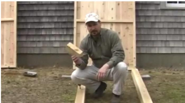
Choose your cedar posts and pick the best end for the top. Use a block or item to be reference for height for all posts. *For Above Ground:* Important tip to remember is to decide how high off the ground you want the kit positioned. Kits are Pre-Drilled.
