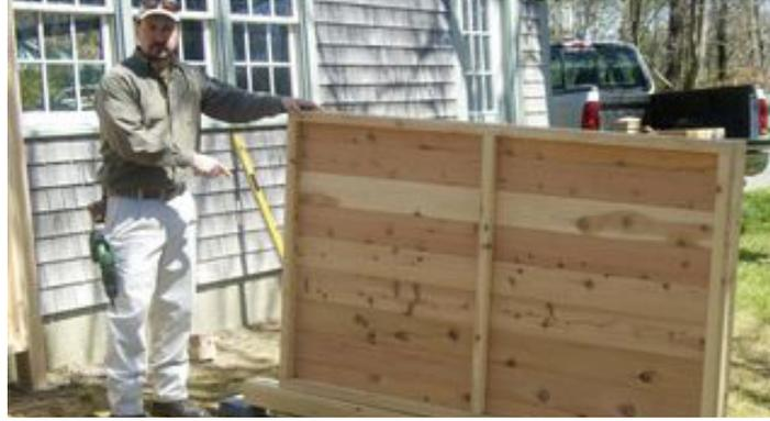
Using Timberloks™ in Hardware Pack, attach a cedar post to large wall. Make sure the rainguard is on top (wider board).
