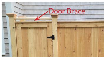
After attaching the door, attach the door brace above, leaving at least a 1/4" space for clearance.
