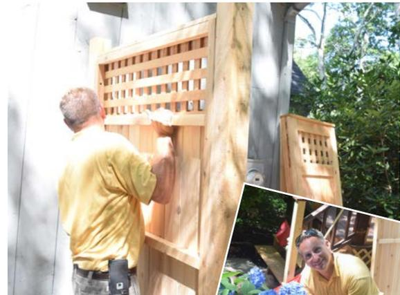
It's that easy. Continue along where the marks are screwing the Timberloks to the posts. This can be done with the assistance of someone.
