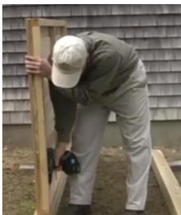
With the Pre-Drilled holes as reference use the Timberlocks™ in your Hardware Pack and connect a large wall to a cedar post. Make sure the inside of the wall is flush to the cedar post. Repeat for the second large wall.
