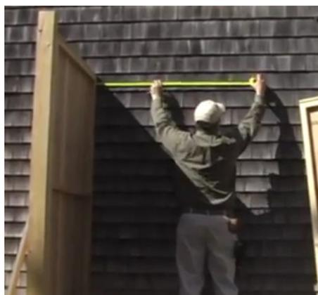
Complete the second wall mount. Make sure the distance from the 1st wall mount is the right size (size of the wall panel) and level. Use a reference point against the wall or mark of with a pen / marker.
