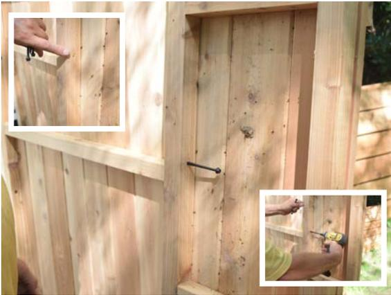
Do the same for the door and small wall. Use the pre-drilled holes as a guide.
