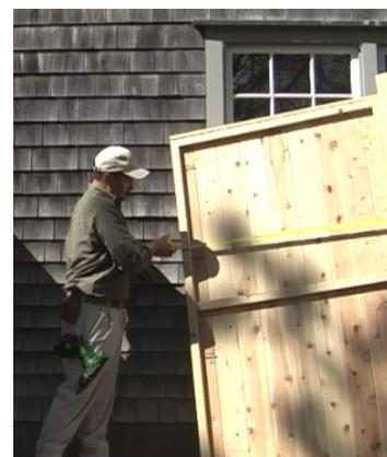
Next, attach one wall to the house. Always making sure the wall is level. Then, measure one of the walls as reference to use for the space along the back side of the house for house mounting.
