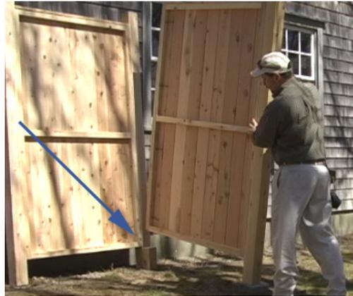
Blue line shows a block to aid with install of 2 large walls.
