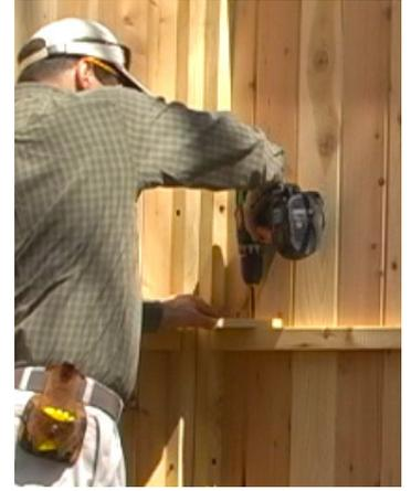
Take the small wall and attach a cedar post to it - again making sure the height from the ground matches the other 2 walls. Add the small wall.
