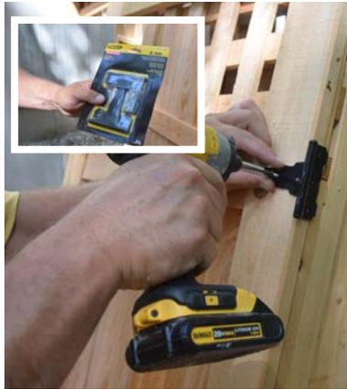
When assembling the door, use hardware supplied and double check the distance on top/bottom to insure good spacing and symmetry.
