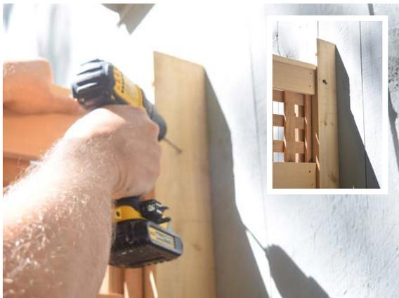
Drill with screws at an angle into the house. You can use Timberlok screws and go about 45 degrees.
