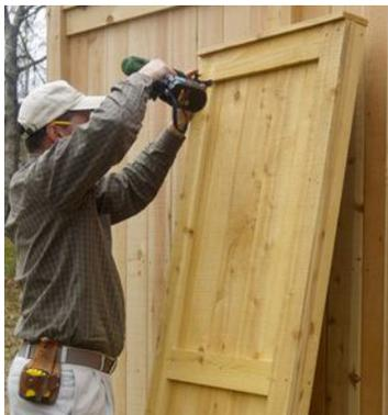
Installing the Door: Use the hardware from the Hardware Pack and install on the door first. Then install the door. Keep about 1/4" between of each side of the door and the shower kit when securing the door.
