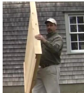
Our walls are built with rain guards. These will be the wider boards of the structure built in to the top of the wall. This part of the wall will be the top.
