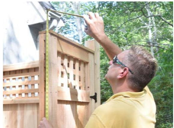
Attach the door to the 1st wall making sure to check that it is level. Adjust the door distance from post as needed on the swing space in between post and edge of door. Allow at least 1/4" clearance on all sides.
