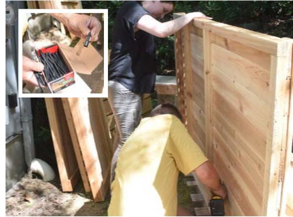
Note: You can adjust the height along the post and all must be that measurement. Use our timberloks provided in the boxes.
