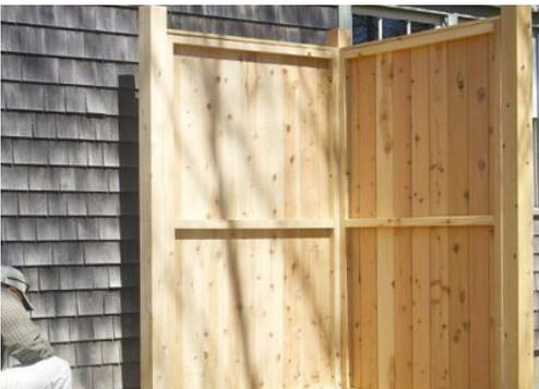
Always make sure inside of panels are flushed to inside of the post.
